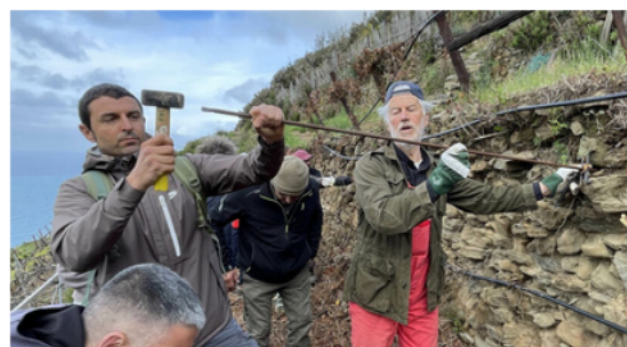
Source: StoneWalls4Life project.
